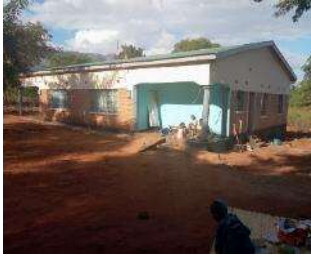
Completed Teachers houses
